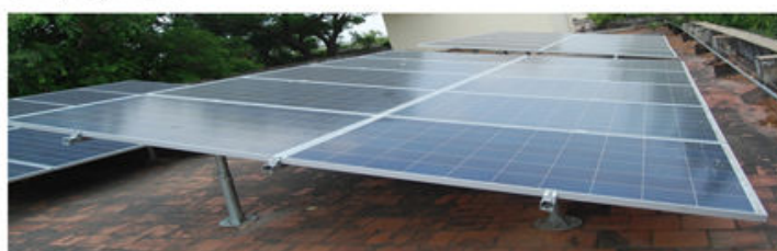
Installation of Solar Power Plant 22.5 KW funded by RUSA and SSS
